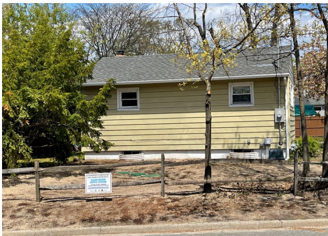
Figure 1: Fuji System installed on a small lot in Bayville
